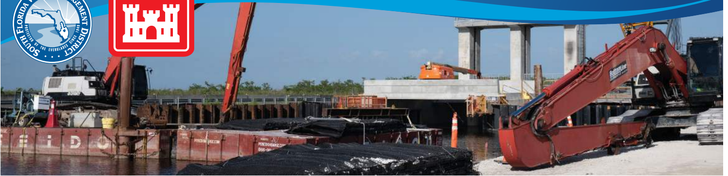
Construction at the Blue Shanty Flow Way.
