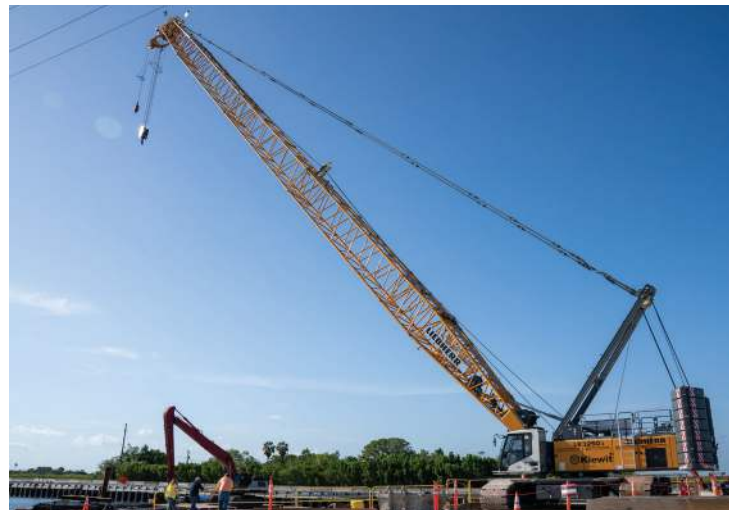
Construction at the Blue Shanty Flow Way.
